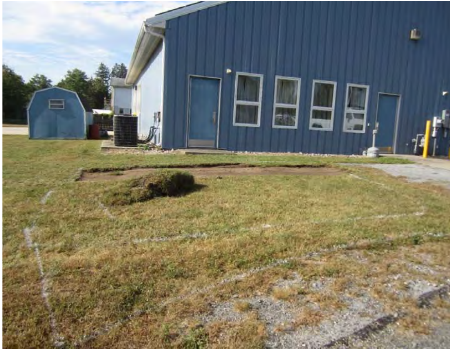
Before, Elmer Ambulance Corps, 30 Broad Street, Elmer, NJ
